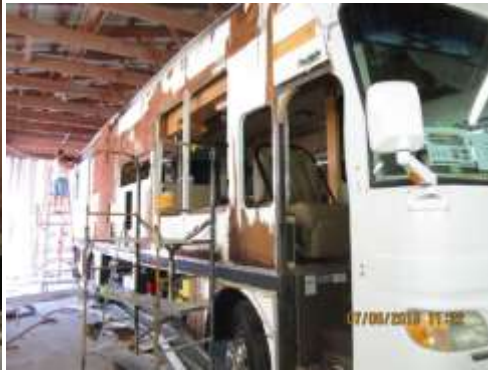
Most passenger side skin removed
